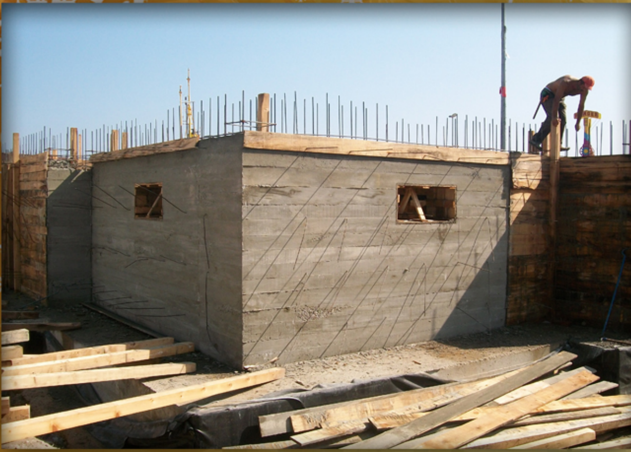
BETON BODRUM DUVARI
